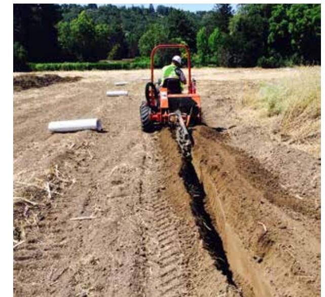
Excavating trench for AMX-T
