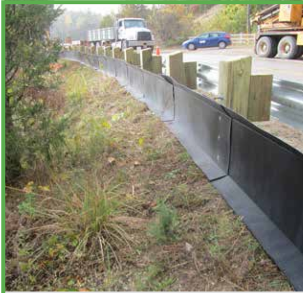
AMX-SP Scored plastic (HDPE) Attached to guardrail
