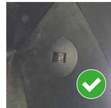
Washer and plastic tie connecting AMX-T sections tightly
