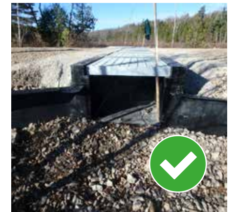
Clean AMX-SP connection to an under-road crossing
