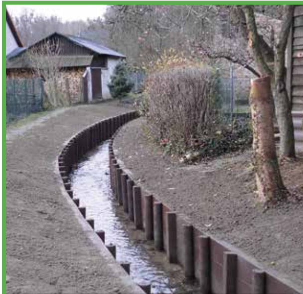
AMX-PL Recycled plastic lumber Retaining wall
