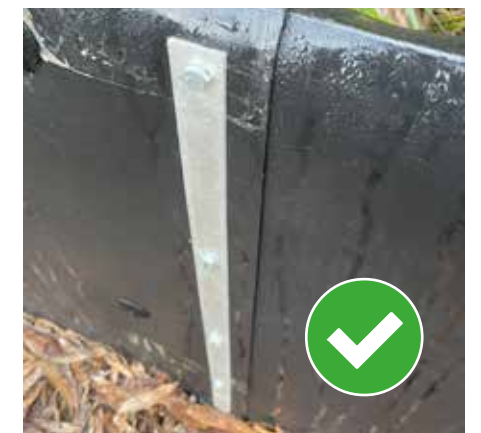
Additional metal strip added to sandwich AMX-SP sections
