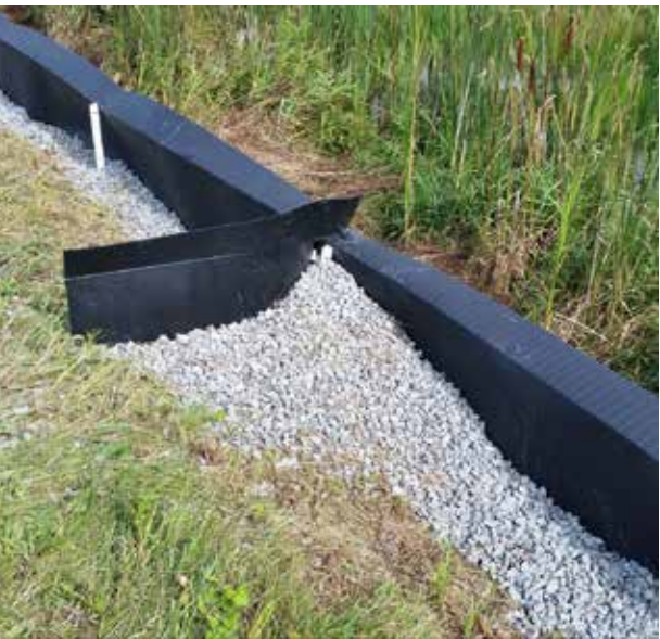
RAMP Gravel ramp over AMX-SP
