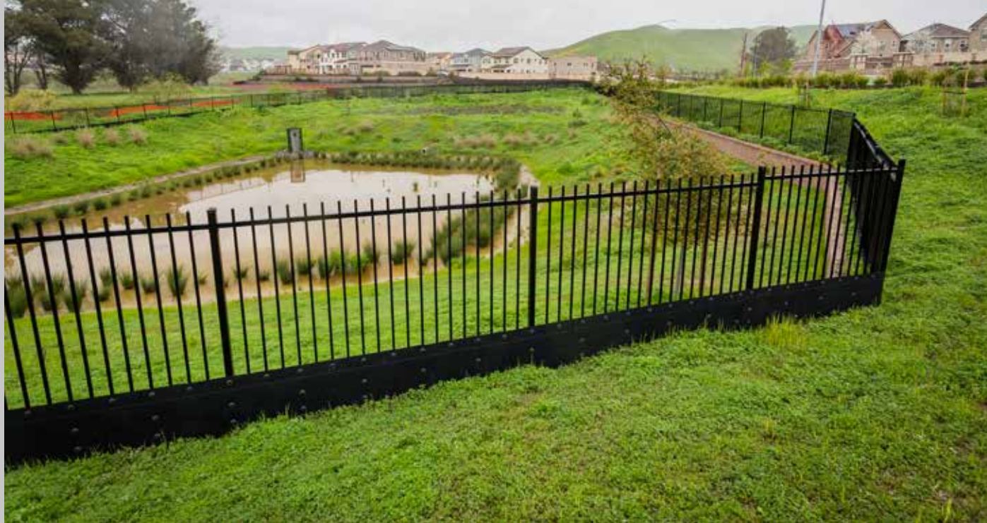
AMX-SP Attached to existing fencing © Travis McCleary
