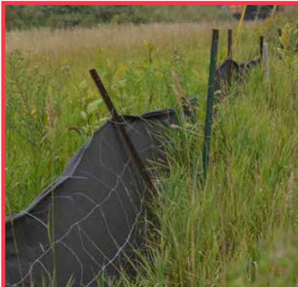
Wire reinforced silt fencing Various species
